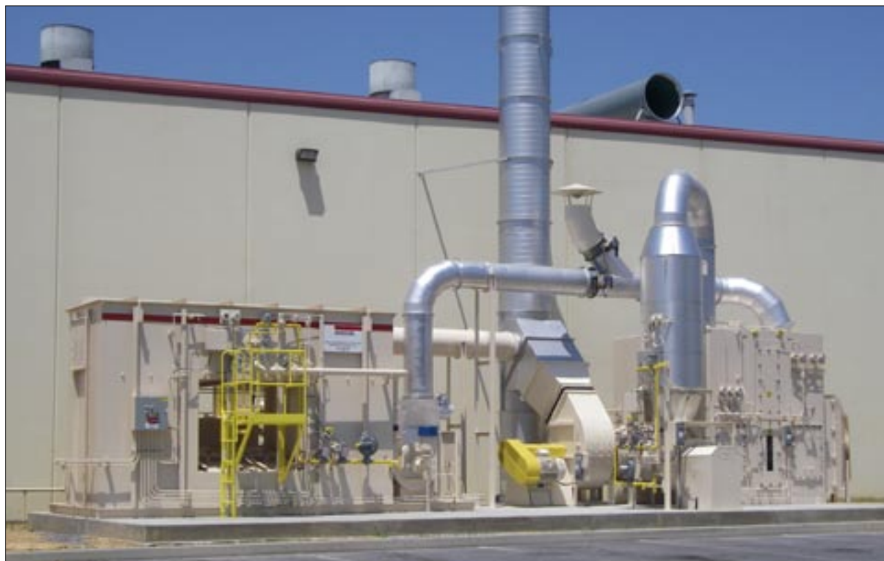
Above and below: Concentrators reduce the air volume being sent to an oxidizer, increasing the capacity and efficiency of an oxidizer system. Courtesy of Anguil.
