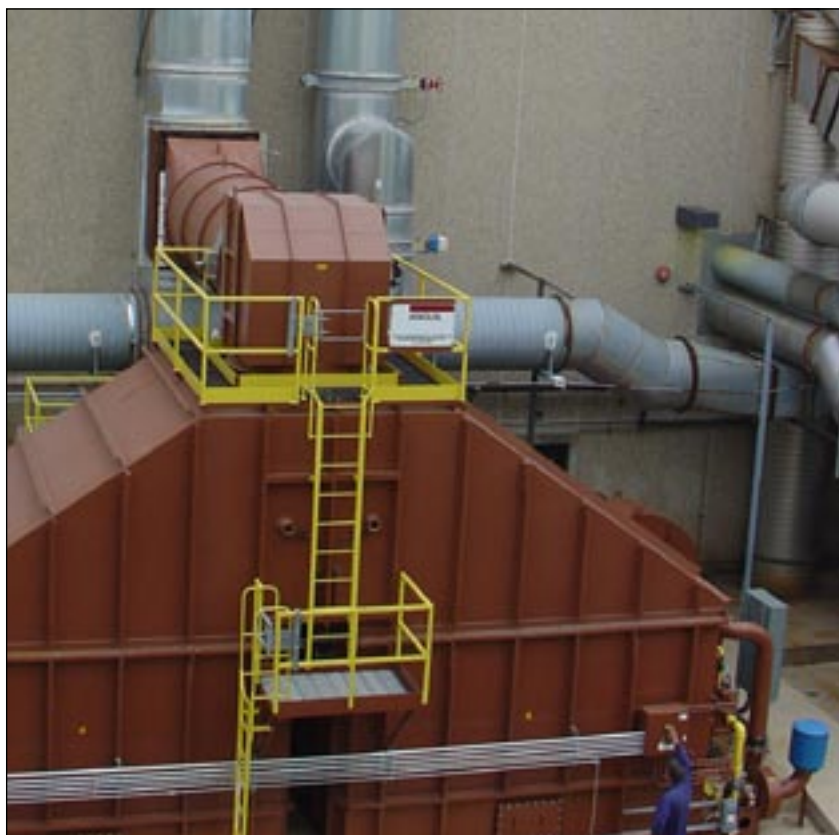
Above and below: Concentrators reduce the air volume being sent to an oxidizer, increasing the capacity and efficiency of an oxidizer system. Courtesy of Anguil.
