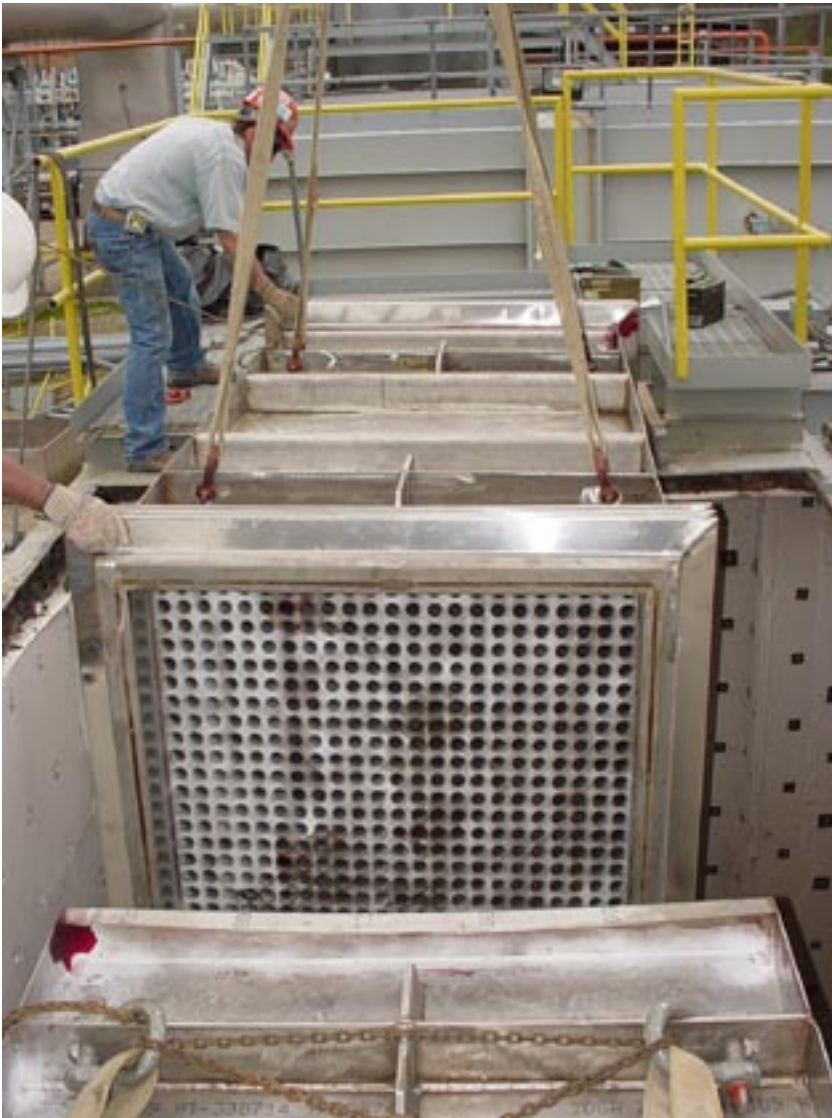
Metal heat exchanger replacement. Courtesy of Anguil.
